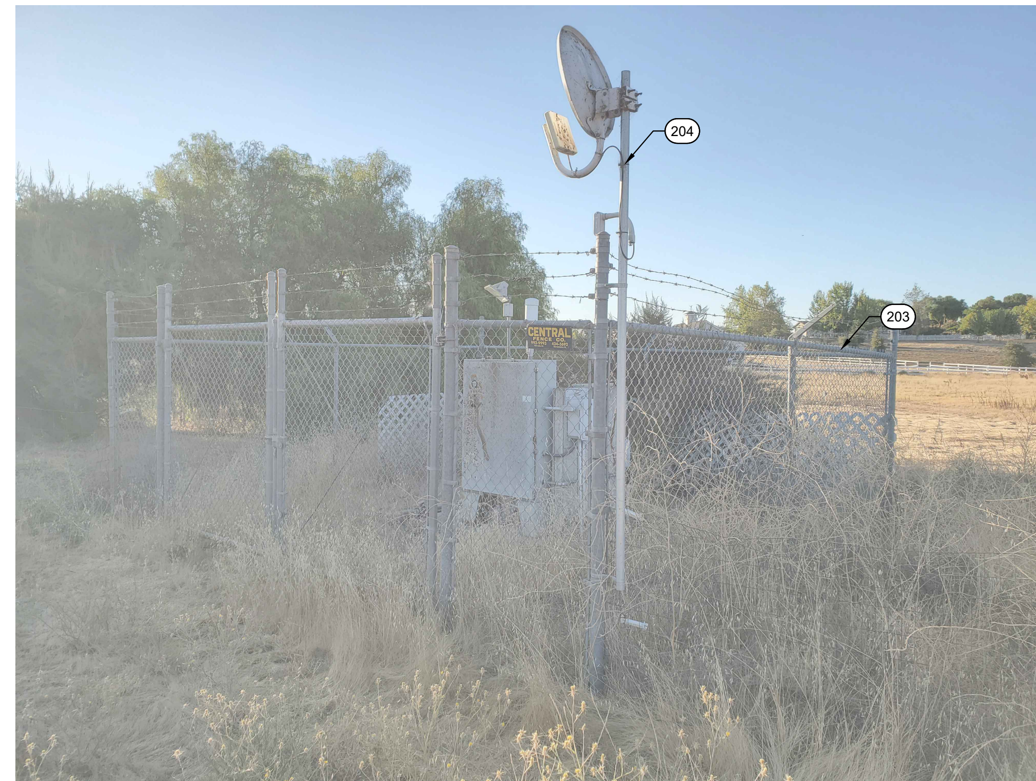
1 WELL SITE 1 ABANDONMENT PHOTOS AND DETAIL
